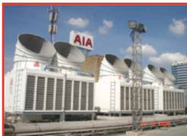
CROSSFLOW TYPE CMS - 500 x 3 SETS AIA TOWER
